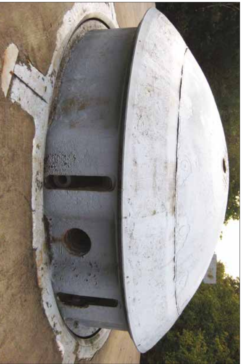
Retractable, rotating cupola with 75mm guns.
