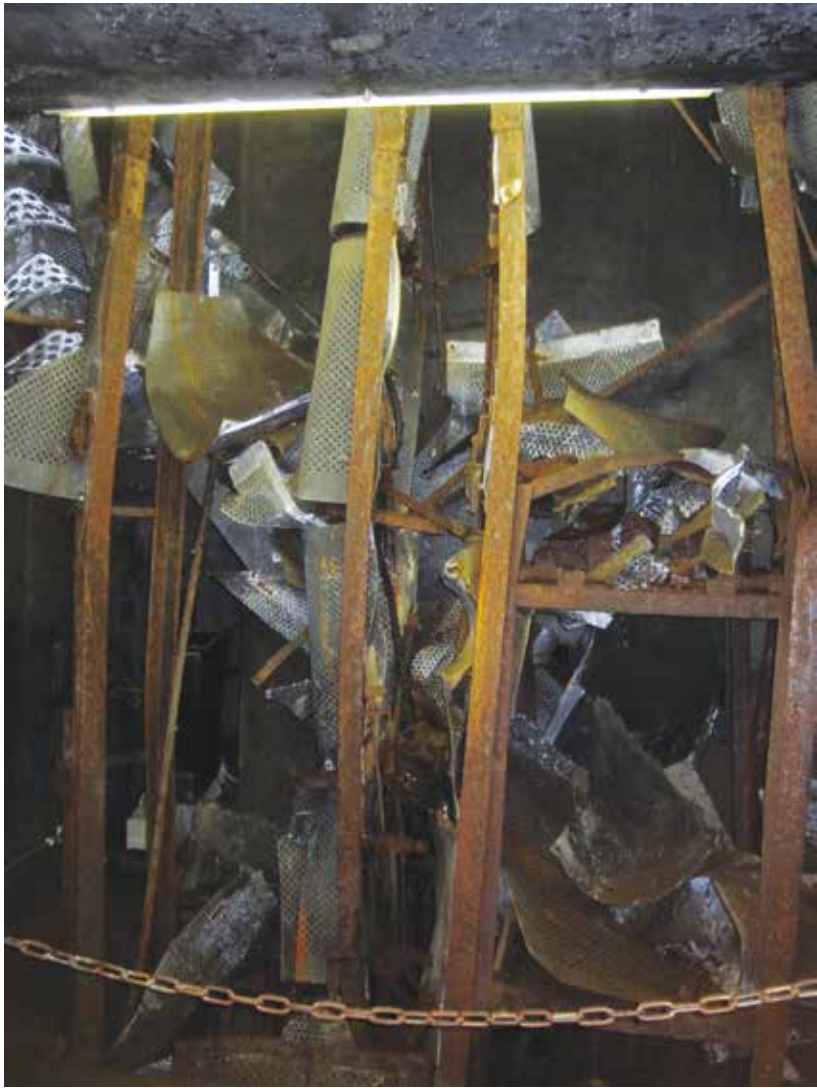
The damage caused by a demolition charge thrown down the elevator shaft.
