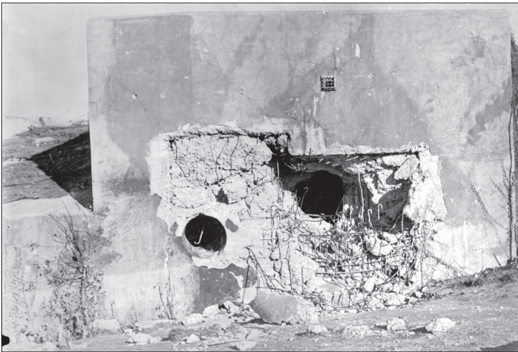
The effects of the Hohlladung (shaped charge) on a Eben Emael gun emplacement.
