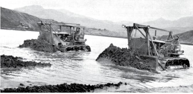
*Bulldozers dredging sand from Adak inlet to use as fill for the new airstrip. The ability of the U.S. forces to construct airfields in the Aleutians was a major factor in defeating the Japanese forces on the islands.*
